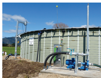
Submersible Stirrer and Above Ground Lifting Frame on KlipTank.
